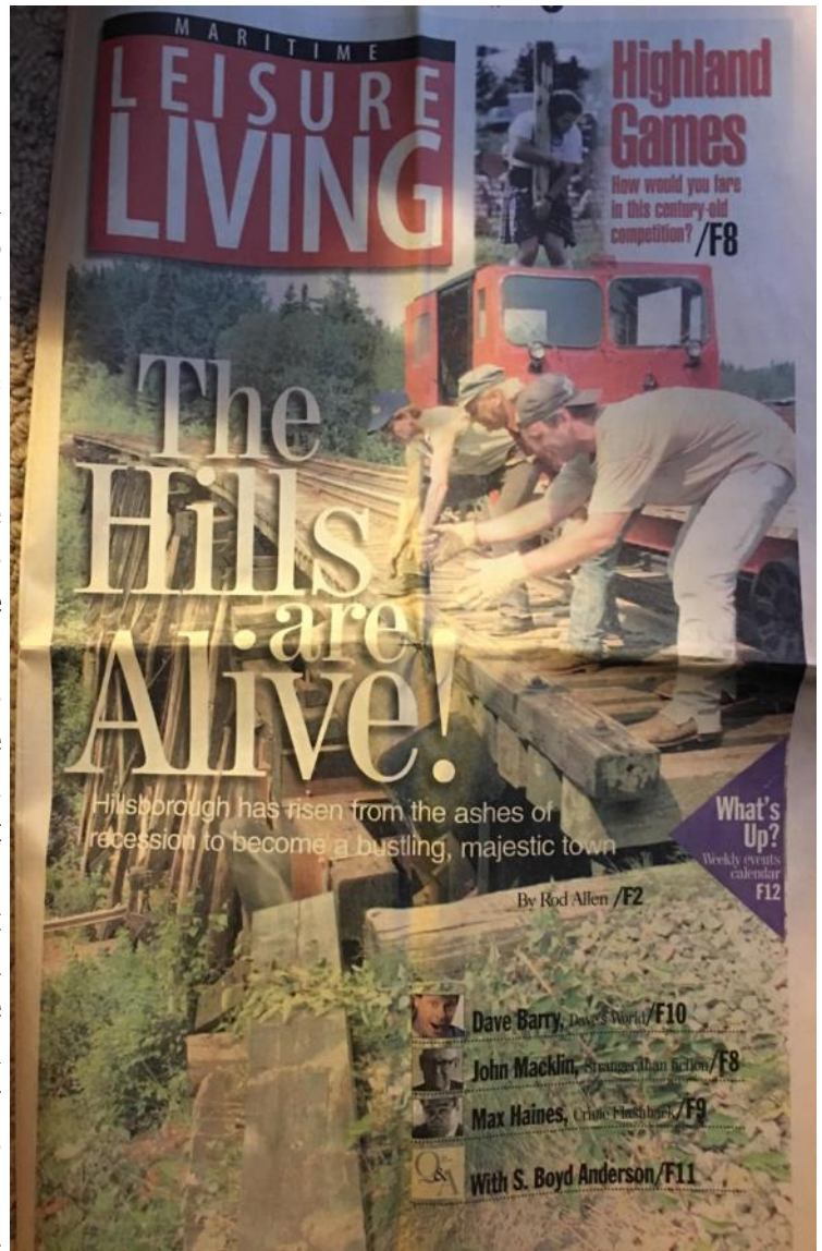
July 25, 1984. Image of the crew working on the Hiram Trestle. The cover reads "The Hills are Alive! Hillsborough has risen from the ashes of recession to become a bustling, majestic town."
